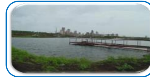
Waste water utilization Pond
