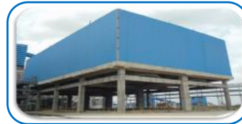
Air Cooled Condensers - TPP
